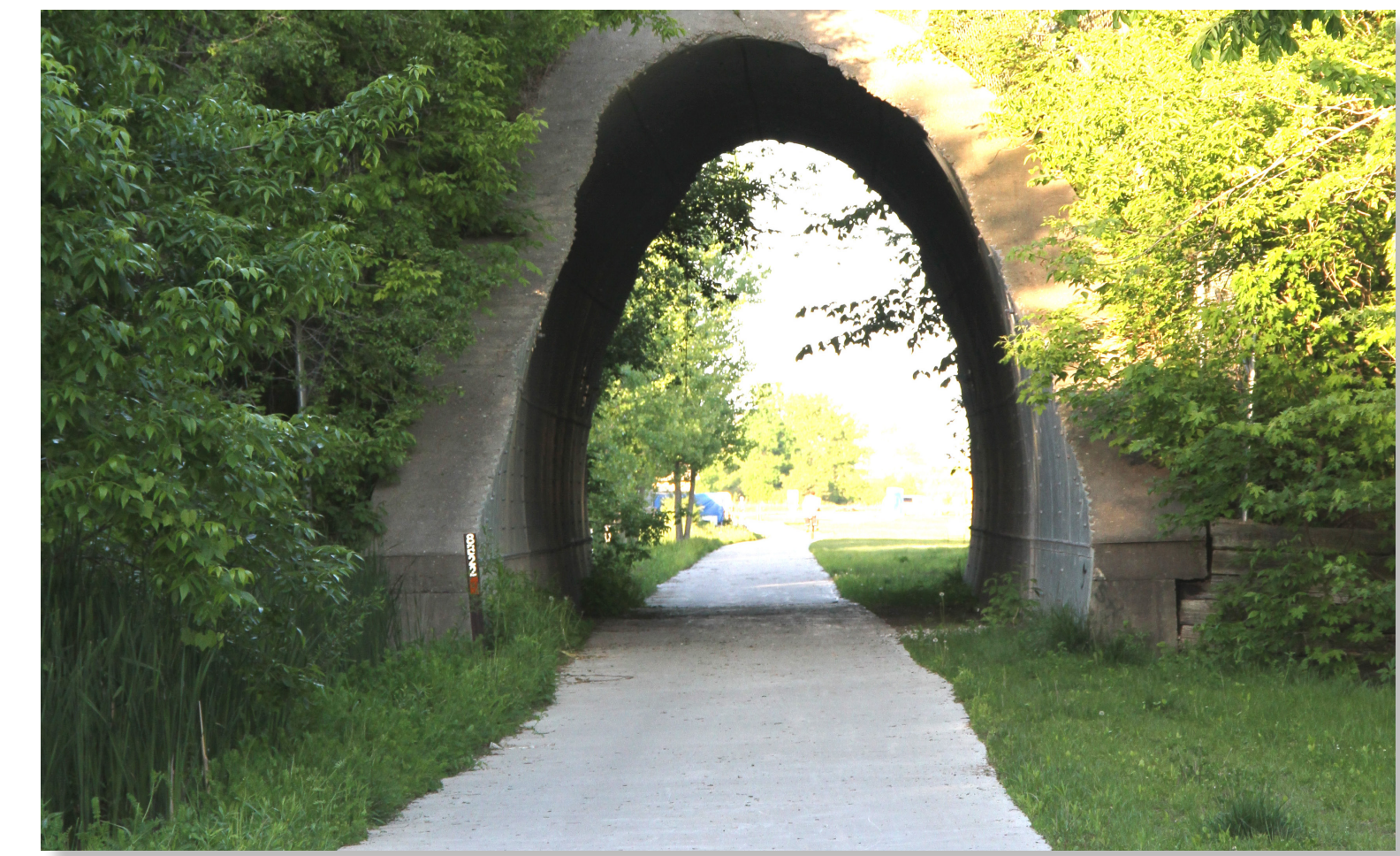
High Trestle Trail. Source: Mary Swalla Holmes
